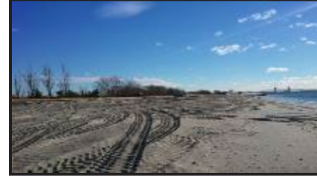
Plumb Beach: 133,000 CY
