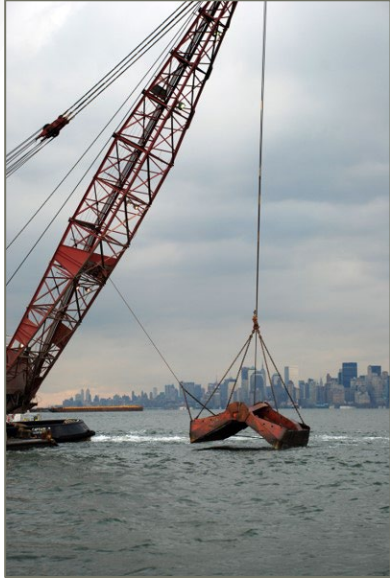
Clamshell - mud, sand, gravel, rocks, and debris
