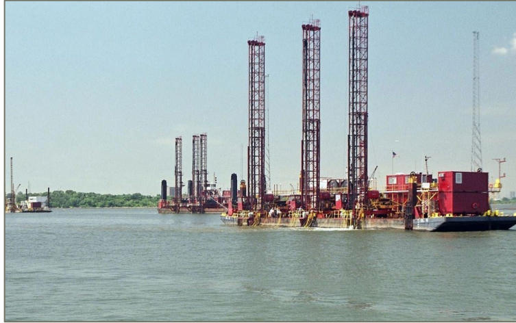
Drill Boats – placing charges for rock blasting
